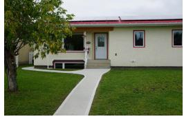
from grade level to the roof with straw bales, which absorbs more greenhouse gas than is required to plant, harvest, and transport.
