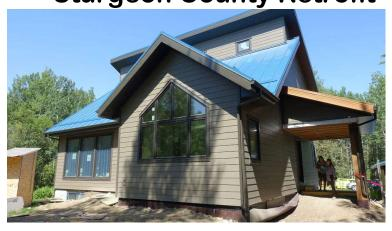
Mostly, the house is planned to be no or very low maintenance and low energy use for the long term on all the major areas. The exterior has cement board siding with a concealed fastener standing seam metal roof to increase fire resistance and reduce future maintenance.
