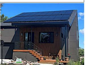
• Net Zero Home – 36-panel solar array (18KW) and efficient heat pump system.
